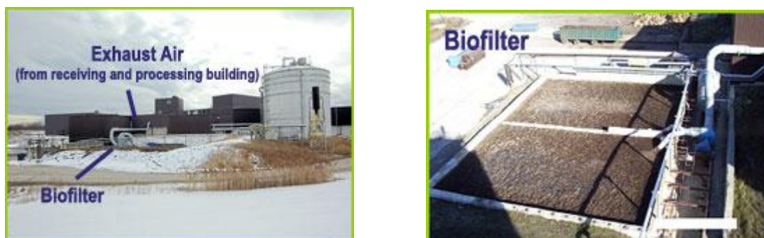
Fig.5.5. Exhaust air from the receiving and processing buildings' ventilation system is passed through a biofilter to remove odour and dust.
