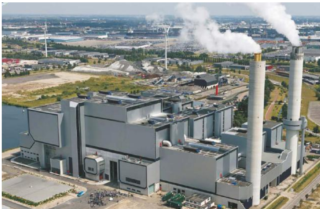
Fot.1.5. The AEB Waste-to-Energy Plant, Amsterdam, the Netherlands
